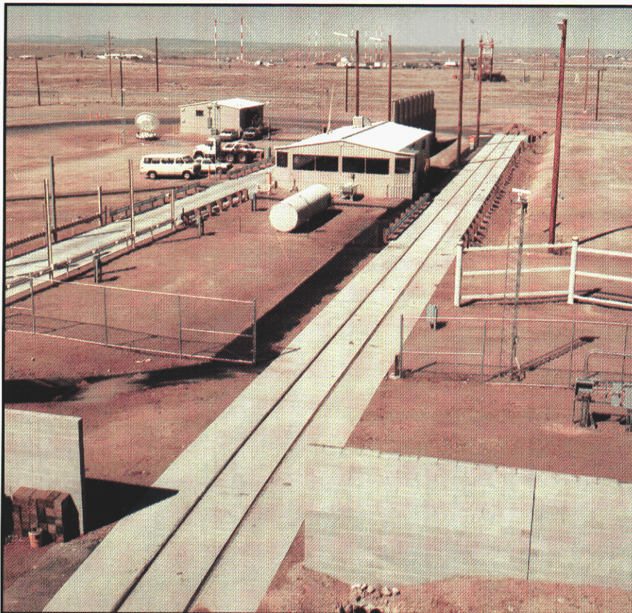
Figure 1. We have constructed a full-scale portal and perimeter demonstration site to show our concepts to government agencies involved in arms control. Two portals are shown: a screening portal through which vehicles too small to contain treaty-limited items may exit, and an inspection portal for inspecting larger objects. The monitored portals would be the only openings in a perimeter fence surrounding a missile production or assembly facility in the USSR. This arrangement is designed to verify that treaty-limited items are not being secretly shipped from the site. The cylinder shows the size of typical objects to be monitored.
