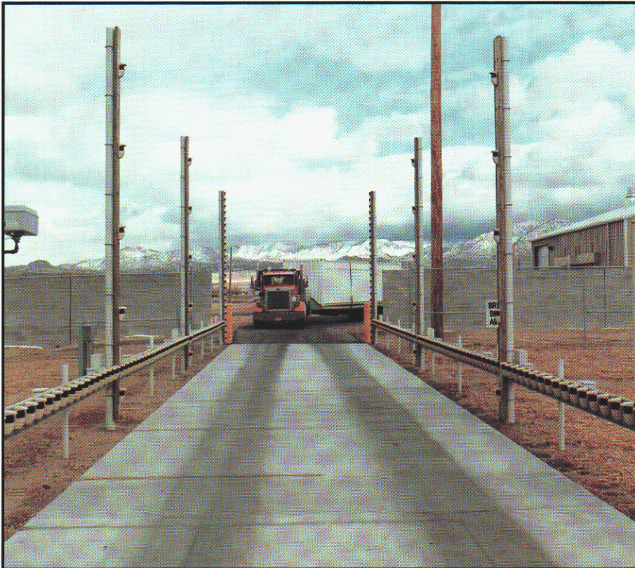
Figure 3. As vehicles pass through the screening portal, they interrupt horizontal and vertical infrared light beams. The profile of each vehicle is then determined to see if the cargo space is large enough to contain a treaty-limited item. All vehicles would be weighed by scales embedded in the roadway.
